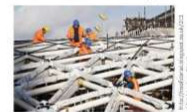
ROOF CONSTRUCTION PROCESS – welding
