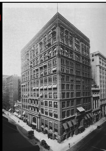
It was completed in 1885 in Chicago, and was the first tall building to use structural steel in its frame.
