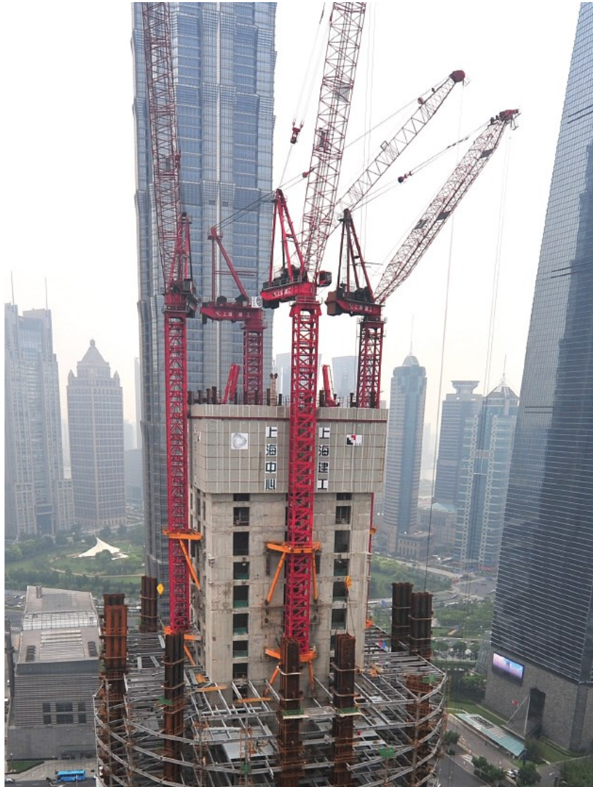
Figure 5.11. Four heavy cranes arranged in the way of out-door handling (Source: Shanghai Construction Group)
