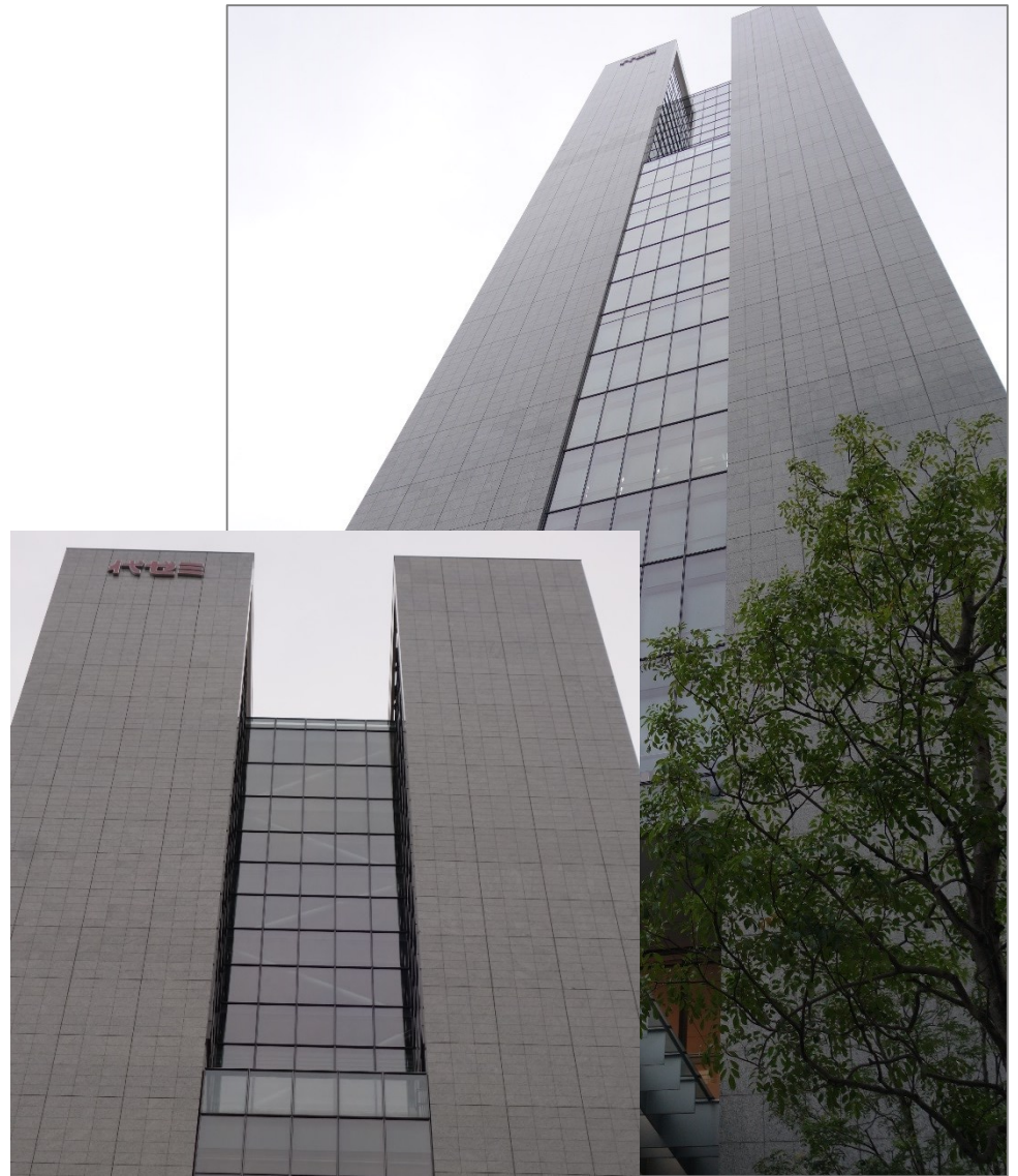
Yozemi Tower Obelisk (2008) – Shinjuku Dampers used in brace configuration coupling two large “mega” walls in short direction for both wind and EQ protection
