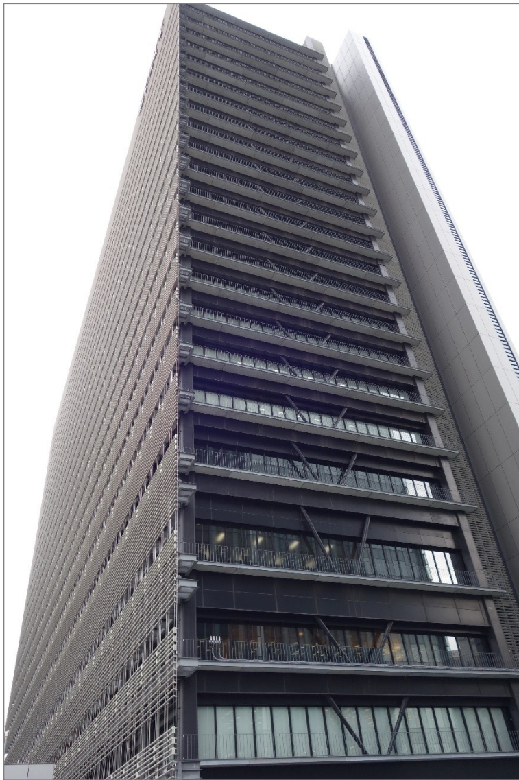
SONY Headquarters (2011) – Shinagawa Dampers used in brace configuration in short direction for both wind and EQ protection
