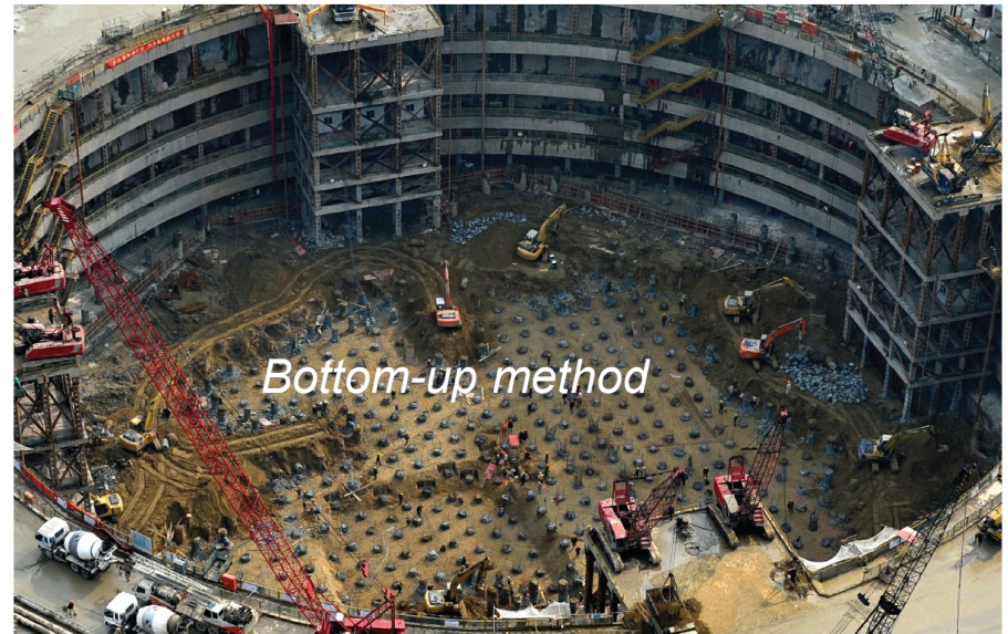
Figure 5.7. Unsupported circular foundation pit of 121 meters' diameter (Source: Shanghai Construction Group)
