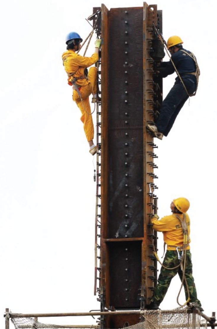
Fixing of mega columns on site. (Source: Ping An)
