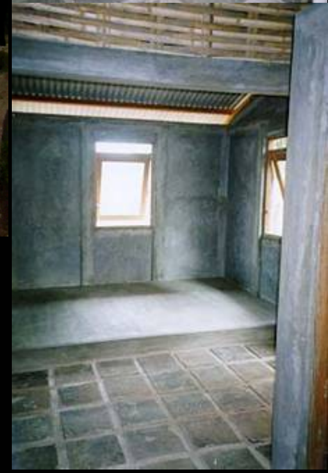
plastered bamboo construction pasir impun - bandung
