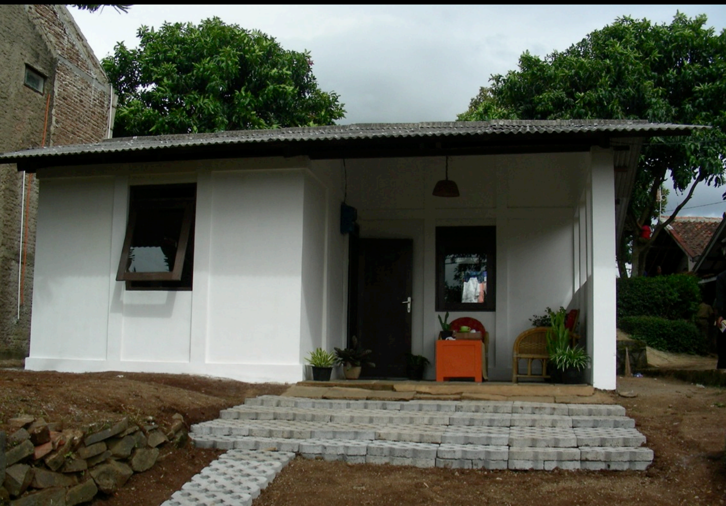
plastered bamboo construction pasir impun - bandung
