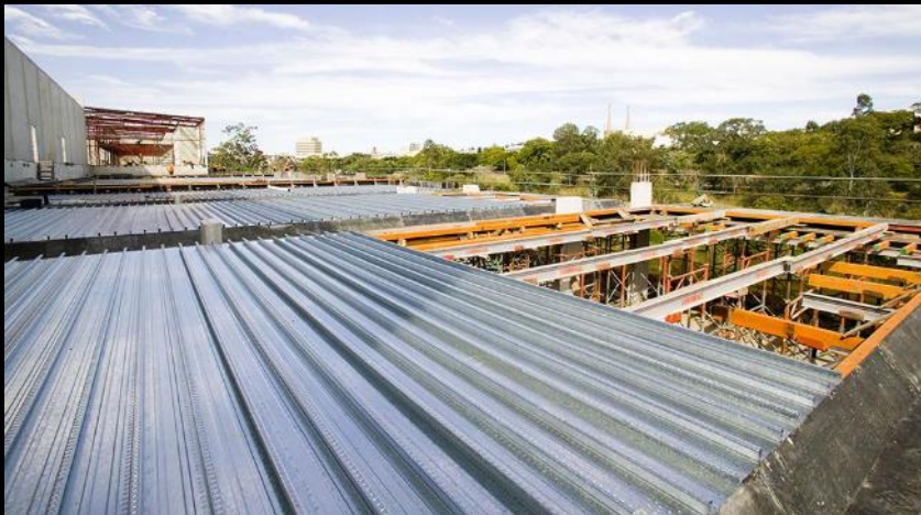
Reinforced concrete slab with metal formwork
