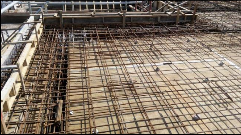
Reinforced concrete beam and slab
